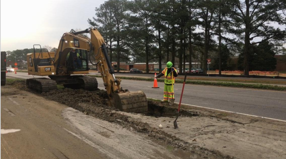
Above: Utility work is a major portion of the Laskin Road Improvements. Over the course of this project, crews will install a total of 3.8 miles of new storm water drainage pipe, 3.1 miles of sanitary sewer pipe and 4.5 miles of domestic water pipe underground. The utility updates are expected to yield significant improvements to storm water management, drainage, and water and sewage systems.
