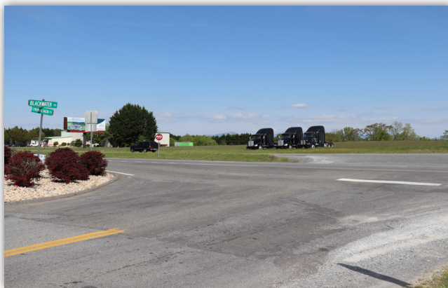
Intersection of Route 460 (Lynchburg-Salem Turnpike) and Route 668 (Blackwater Road).
