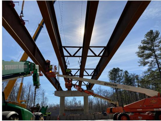
*Photo: Cranes hold steel bridge beams over Route 143 while crews in bucket lifts secure the beams in place.*
