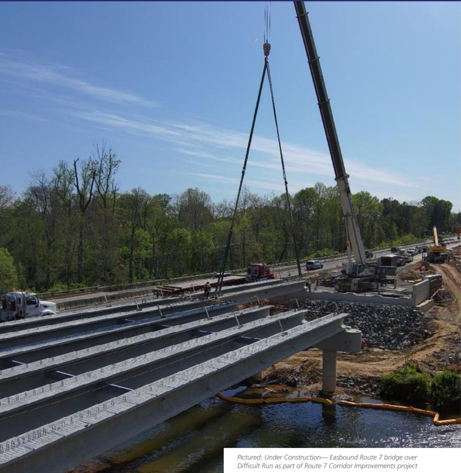
*Pictured: Under Construction— Eastbound Route 7 bridge over Difficult Run as part of Route 7 Corridor Improvements project*
