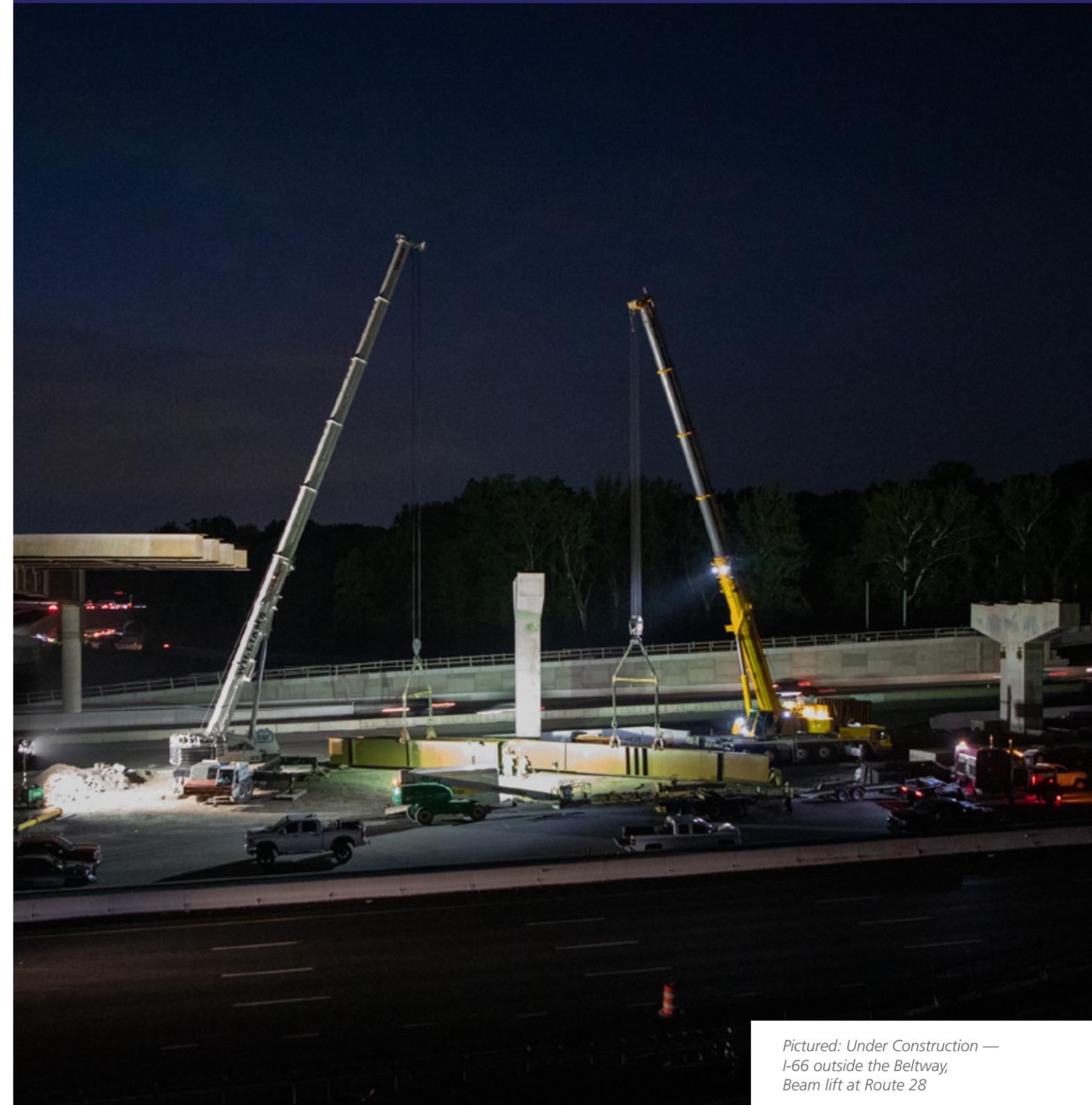
Pictured: Under Construction — I-66 outside the Beltway, Beam lift at Route 28
