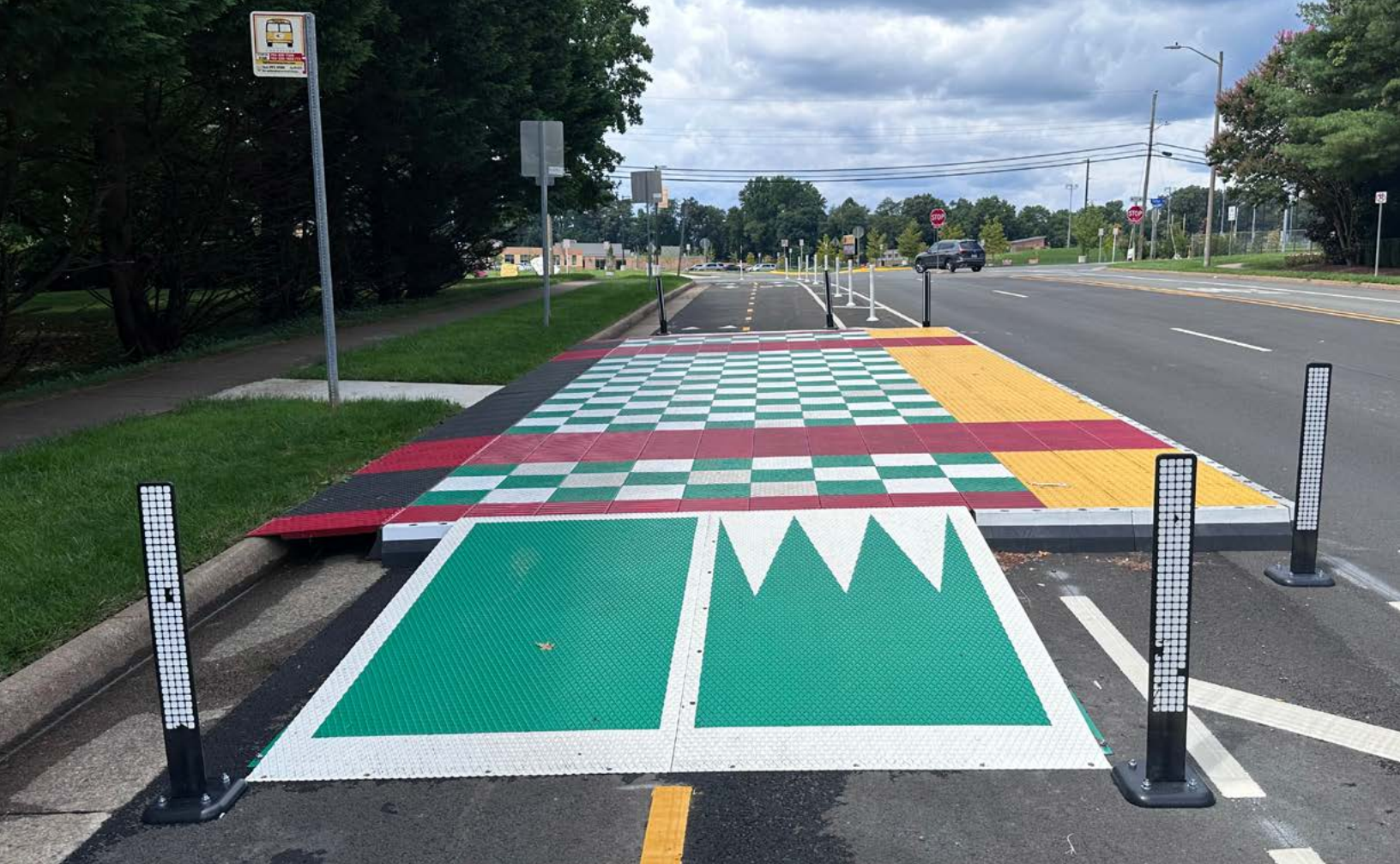
Above: "Zicla" modular bus platform in the cycle track on Country Creek Road in Fairfax County which provides pedestrians a boarding platform to buses in the vehicular travel lane.
