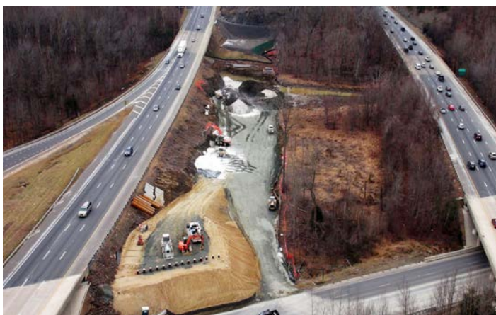
Figure 5: Branch mitigated acid-producing rock on the 95 Express Lanes Project with the use of agricultural lime
