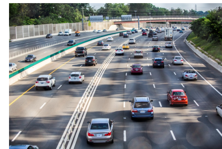
95 Express Lanes retrofitted a two-lane section to three lanes, preserved miles of existing barrier and reduced drainage impacts.
