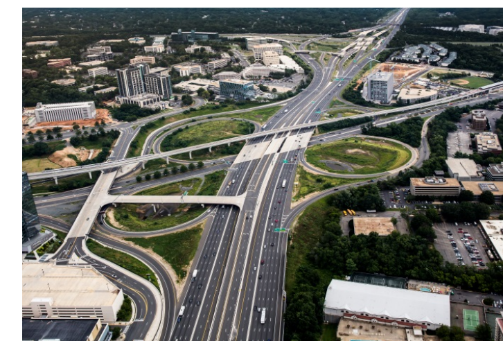
495 Express Lanes involved reconstruction and new construction of highway, roadway, intersections, interchanges and numerous bridges in urban and rural areas requiring attention to soils and maintenance of traffic.
