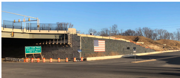
Figure 3.5.5 - Temporary Wire Wall used Route 7/659 Interchange
