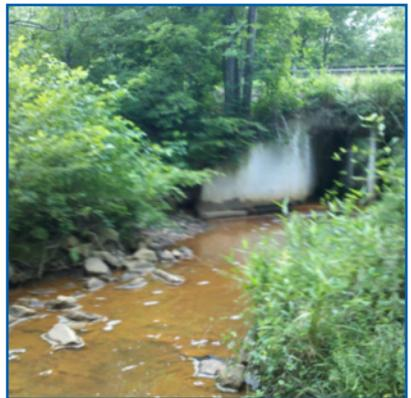
Presence of iron bacteria in culvert, as well as in stream. Note the orange-brown color.
