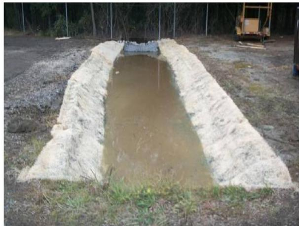
Rock Check Dams and Drainage Ditch Soil Stabilization
