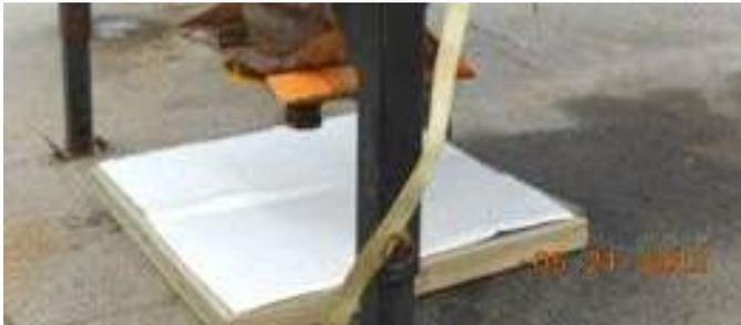
Oil absorbent pad attached to wood frame/pallet
