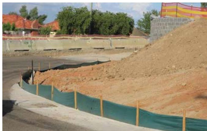
Silt Fence around soil pile
