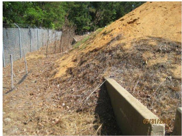
Clean up of sand/erodible materials pushed overtop of jersey-wall control structures
