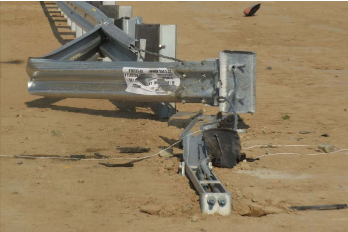
FIGURE 38. Test Article Damage
