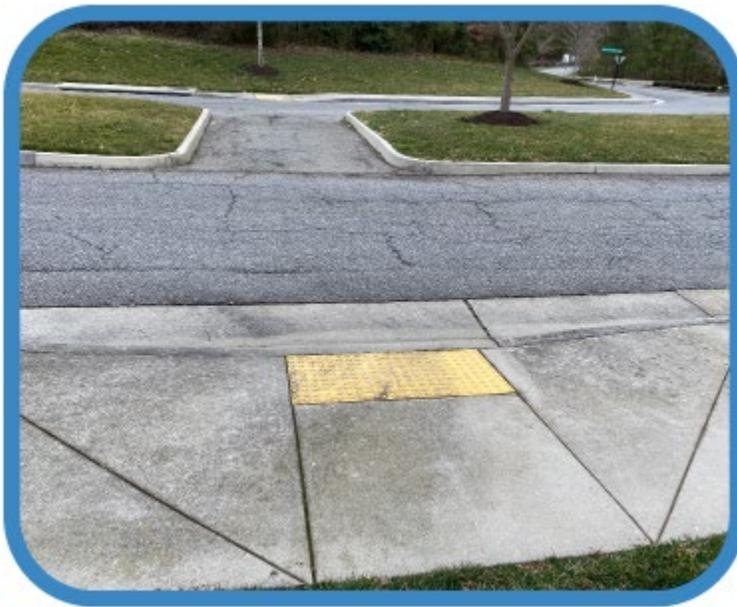
Figure 11 Missing crosswalks at the roundabout
