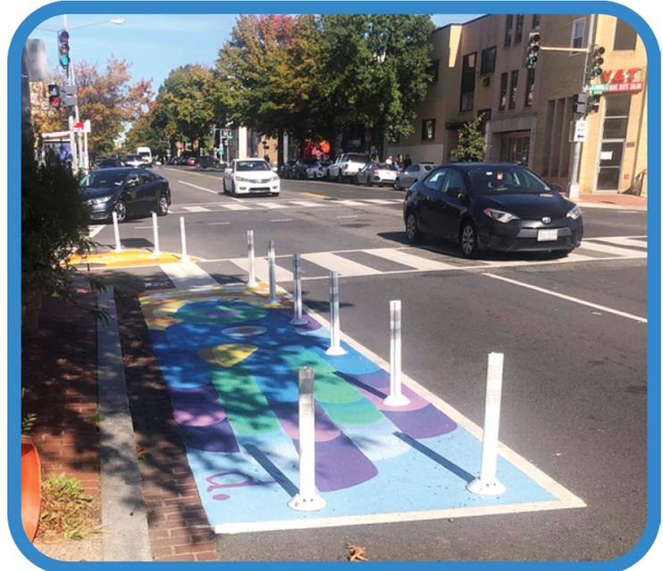
Figure 12. Flex-post curb extensions with paint at a crosswalk in Washington, DC.
