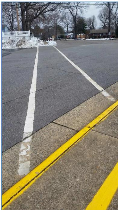
**Figure 6. School property at Cresswell Road (facing east).** Although there are two marked crosswalks at the intersection of school property and Cresswell, neither crosswalk is equipped with curb ramps and the crosswalk on the north side of the intersection (shown here) is quite long (approximately 75 feet).
