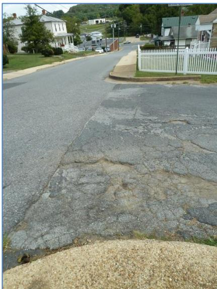
**Figure 3.** Intersection of Gay Street and Bessie Weller Drive, looking east. A lack of cross walks and curb ramps discourages potential walking and biking.
