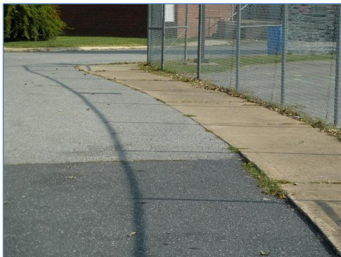
**Figure 4.** The sidewalk along Bessie Weller Drive is level with the roadway at points.
