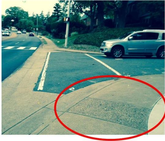
**Figure 3** A single curb ramps serves each corner instead of the preferred one curb ramp per crossing. As a result, the curb ramps are oriented at a diagonal to the crosswalk, forcing pedestrians into motor vehicle travel lanes (i.e., oncoming traffic). The curb ramps also do not meet current ADA guidelines, which require truncated dome detectable warnings.
