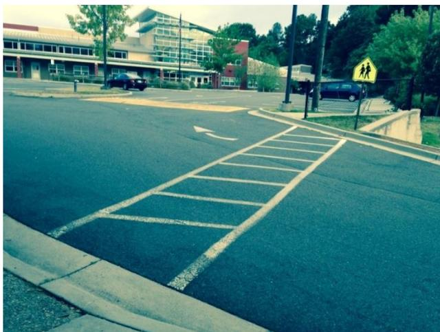
**Figure 10** There is no curb ramp on the north side of the school access drive.
