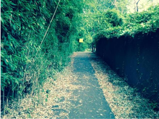
**Figure 12** The pathway connection between Culpepper Street and the school property is covered with debris, and bushes narrow the path's clear width.
