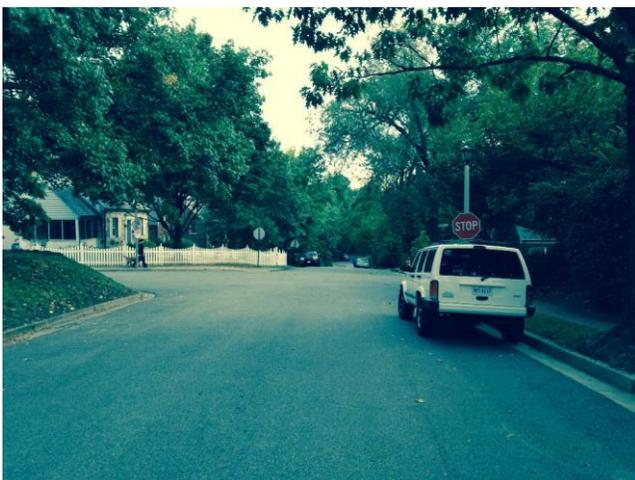
**Figure 8** At the intersection of 18th Street N. and N. Wakefield Street, none of the crosswalks is striped. Consequently, motorists may be less likely to anticipate pedestrians at this crossing. Also, vehicles sometimes park too close to the intersection, making it more difficult for pedestrians and motorists to see each other.
