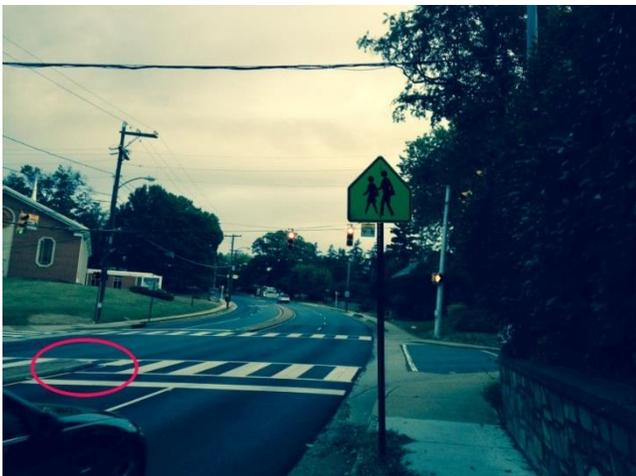
**Figure 2** The concrete median on N. Glebe Road extends into the crosswalk, forcing some pedestrians, such as those with strollers and mobility impairments, out of the crosswalk and into oncoming traffic to navigate around the median nose.
