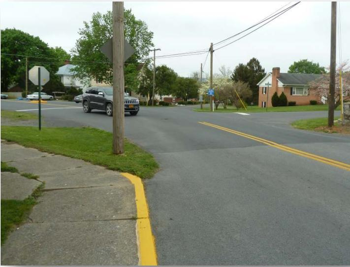
Intersection of Hawksbill Heights Drive/Amiss Avenue and Luray Avenue – on Amiss Avenue looking south. A lack of crosswalks and the irregular intersection geometry can make this crossing uncomfortable for pedestrians. The vehicle in the photo is making a right turn onto Amiss Avenue.
