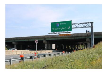
The project is raising the height of the new I-95 overpasses on Route 17 to avoid strikes and damage from trucks and oversize vehicles passing underneath.
