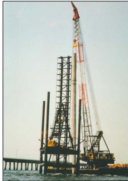
**Figure 6-9: 66-inch Dia. Concrete Cylinder Pile Construction (Chesapeake Bay Bridge Tunnel Project)**
