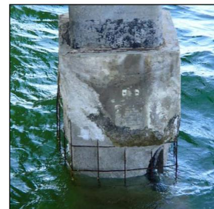
Figure 2-4: Existing Pile Jacket Deterioration
