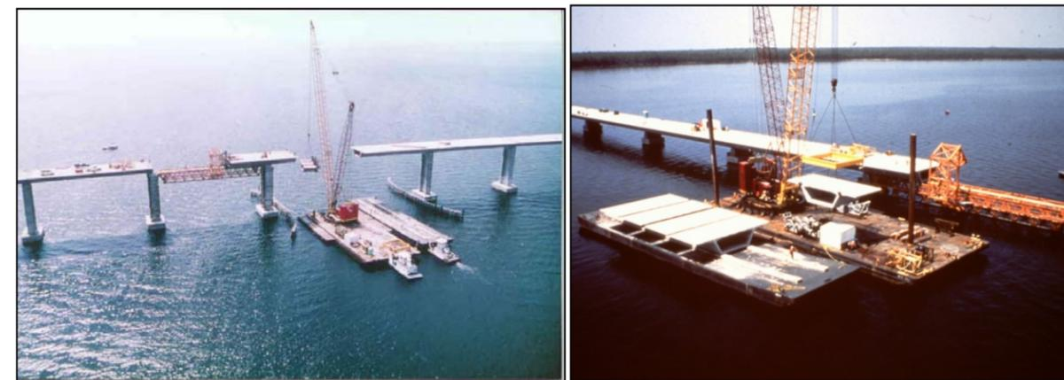
Figure 6-7: Precast Segmental Box Girder Erection Truss
