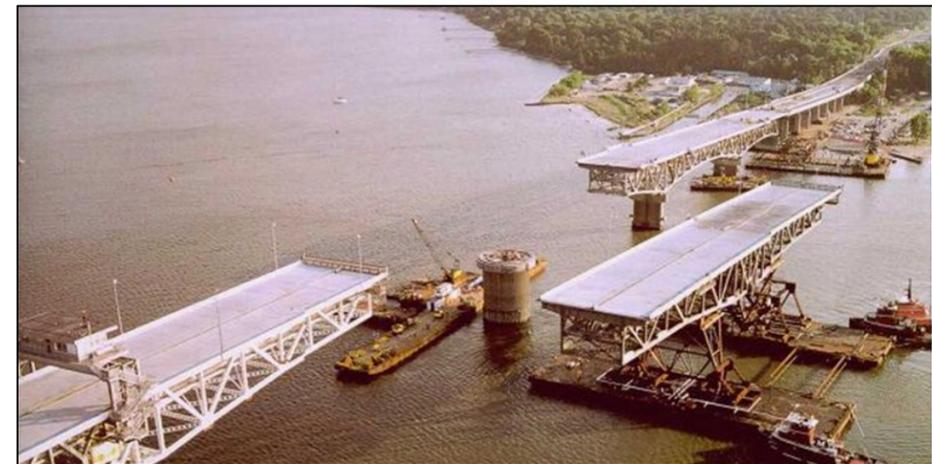
**Figure 4-2: Coleman Bridge Construction: Float In of Swing Span**
