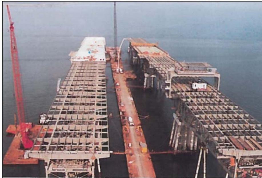
Figure 4-3: Coleman Bridge: Construction of Bridge in Fabrication Yard
