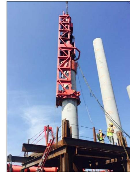
**Figure 6-10: 54-inch Dia. Concrete Cylinder Pile Construction (Bonner Bridge Replacement Project)**
