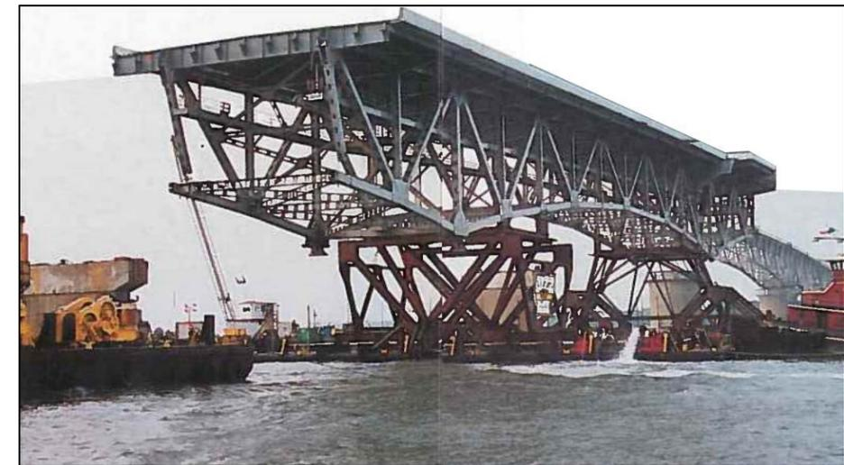
Figure 4-5: Coleman Bridge: Float In of Anchor Span
