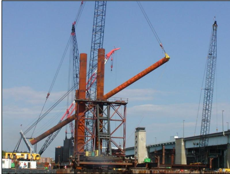
Figure 6-11: Woodrow Wilson Bridge over the Potomac River, MD (72-inch Dia. Steel Pipe Piles)
