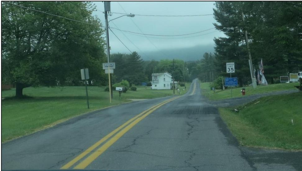
As shown in the pictures, the posted speed limit along Reservoir Road is 35 mph and there are very narrow lanes. Any cyclists must travel on the roadway in mixed traffic, meaning there is no buffer from the travel lanes. Figure 17 shows the four levels of traffic stress with LTS 1 being the most comfortable for all ages and abilities. The existing conditions along Reservoir Road indicate the least comfortable LTS 4.
